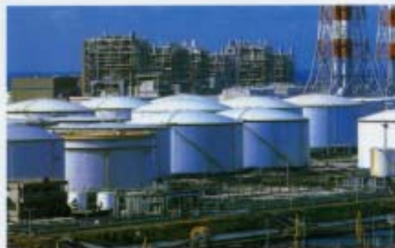
化學、染整廠 CHEMICAL DYEING PLANT
